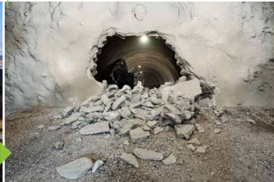
May 2024 Breakthrough of the Lokev Tunnel – Slovenia's longest tunnel was excavated
