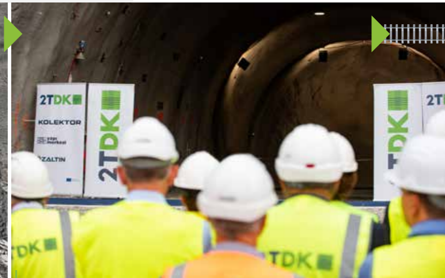
June 2022 Breakthrough of the first tunnel
