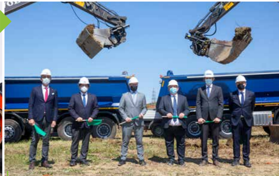
May 2021 Start of main construction works
