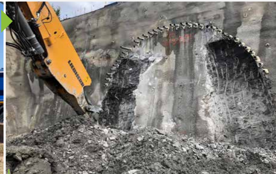
September 2021 Start of tunnel excavation
