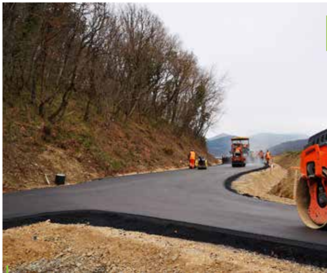
March 2019 Start of construction of access roads
