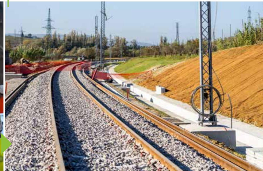
October 2024 Start of track laying
